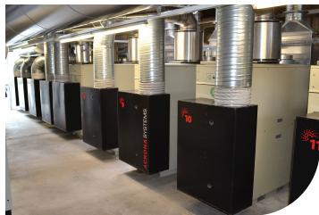
Twelve CR65 Capstone microturbines installed in a CHP application at the Gefu Produktions AG manufacturing facility in Lucerne, Switzerland, use milk sugar from the manufacturing process to generate onsite electricity and heat.
