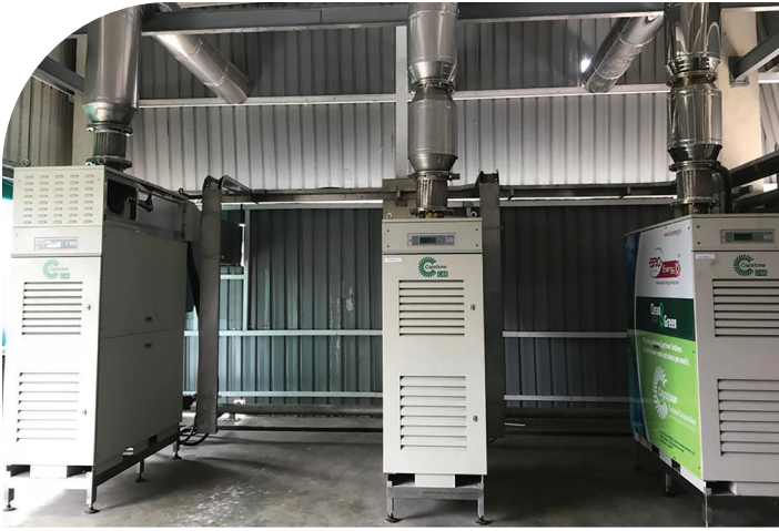
Three C65 microturbines provide power to the India-based dairy conglomerate helping them meet government regulations while also providing them reliable power and reducing energy cost.
