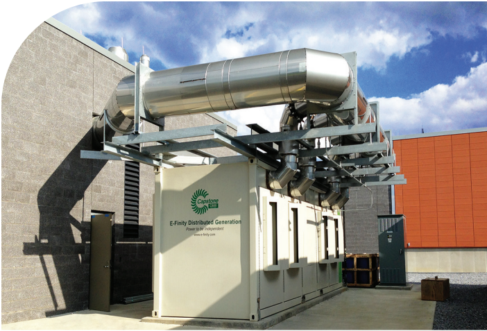
A Capstone C800 microturbine operating in a CCHP application producing 800kW of clean and reliable power for the PSECU data center UPS.
