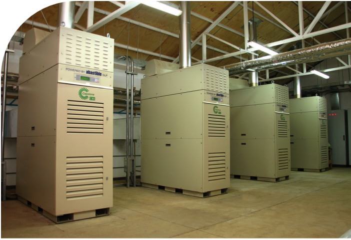
The cogeneration system supports 100 percent of power demand for this luxury hotel and is capable of delivering 1,752GWh of electricity and 3,504GWh of thermal energy per year at full load.
