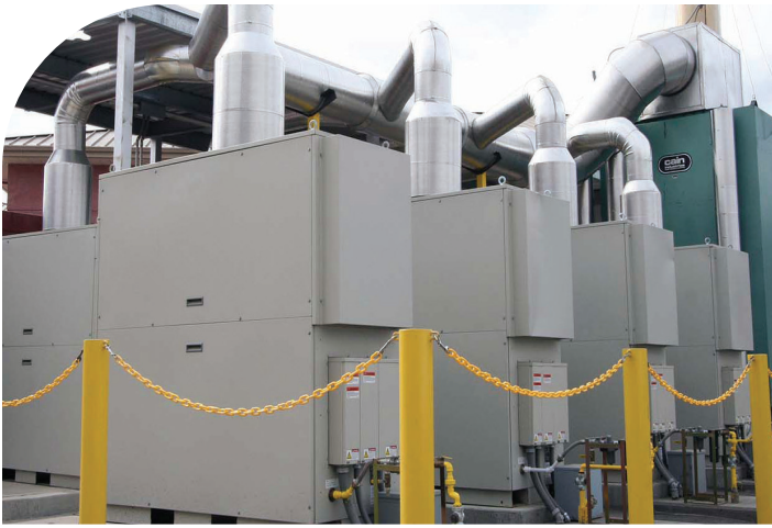
Eight Capstone C60 microturbines provide combined cooling, heating and power to EMWD's Operations and Maintenance Center in Perris, California, while a ninth microturbine provides combined heat and power to the
