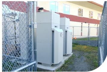
Two C65 ICHP microturbines provide all of the medical facility's thermal and electrical needs, decreasing their carbon footprint by more than 70% and reducing noise pollution.
