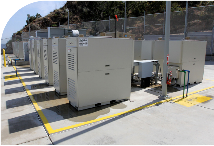
23 Capstone C65 microturbines provide prime power to Southern California Edison's Avalon site on Catalina Island.
