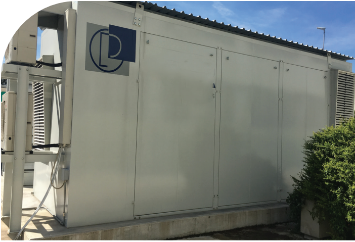
Two natural gas-fueled C200 microturbines, along with a rotating UPS and emergency generator, combine for a clean and reliable CHP microgrid for the nutrient production facility.
