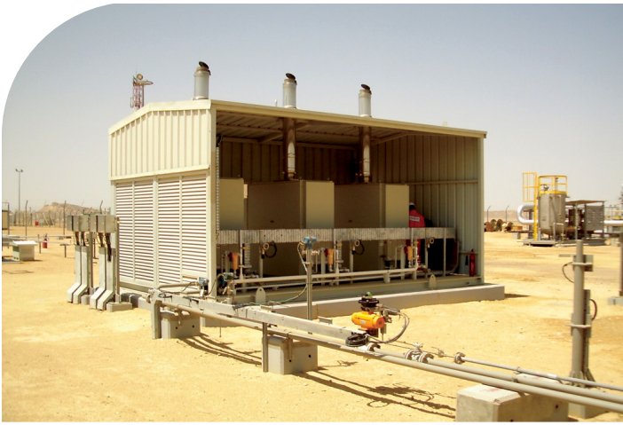
Three C65 Capstone microturbines provide prime power for the remote oil and gas site. The microturbines have run continuously for more than 24,000 hours, providing 95% uptime.
