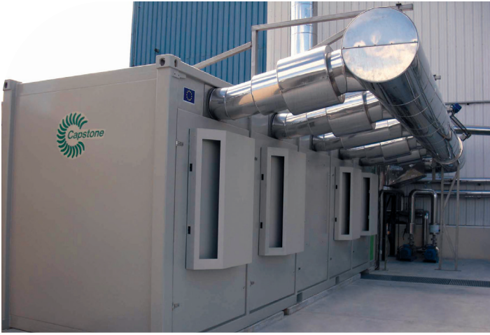
A C800 Power Package is fueled by methane from the treatment of sludge waste (from grape skins and stems) following the distillation of wine to make Cognac.
