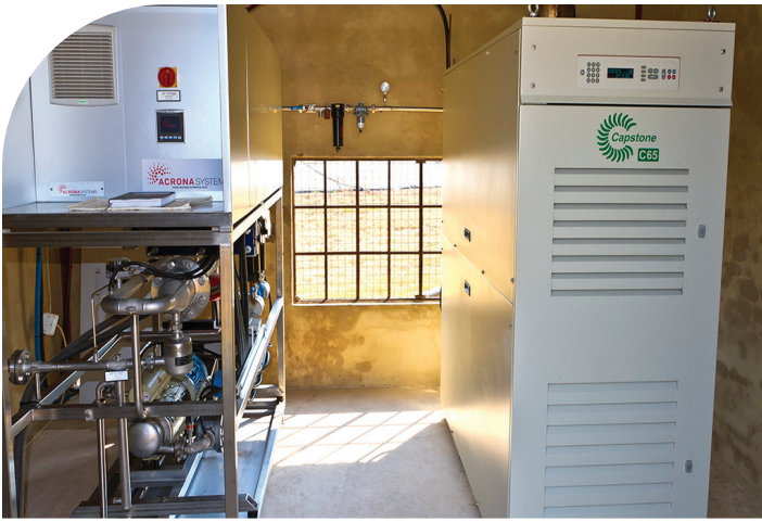
A digester gas-fueled Capstone CR65 microturbine provides power to Swineline Farm in South Africa.
